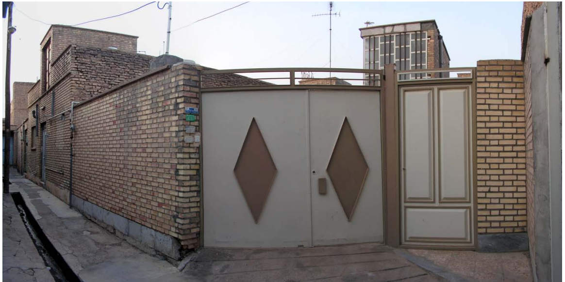
Figure 8: Main entrance of old building which was chosen for demolition
