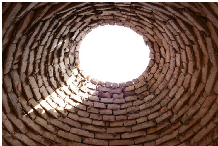
Figure 7: Catenary-shaped domes for improved ventilation and natural cooling (urbanNext, 2024)
