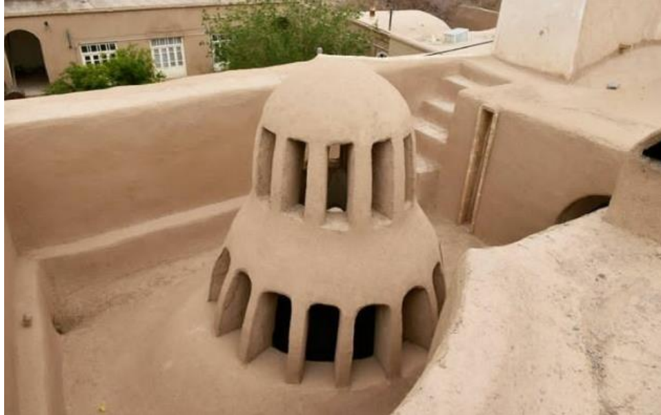
Figure 30: Natural Ventilation Structures of Houses in Mehriz Village
