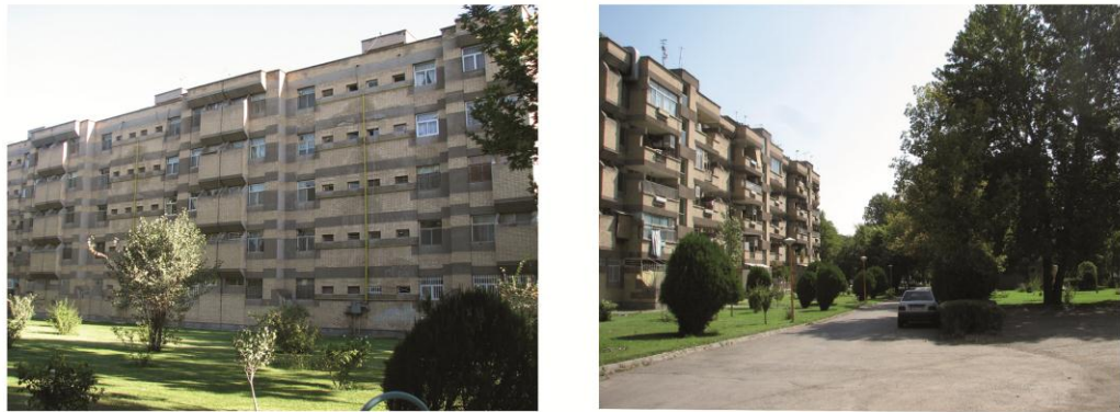
Figure 16: (Left) backside of blokes (Right) green spaces in front of blocks,(by author)
