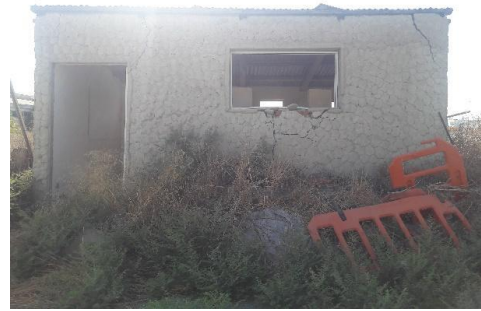
Figure 3.121: Wall Cracks (Author)
