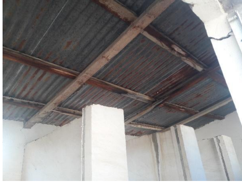
Figure 3.120: Roof Damages (Author)
