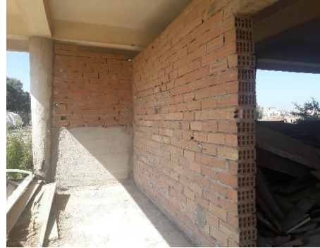
Figure 3.43: Brick Wall Additions on Ground Floor of Offices (Author)
