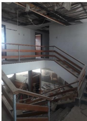
Figure 3.74: Collapsed Suspended Ceiling (Author)
