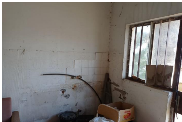
Figure 3.109: Loss of Ceramic Tiles in Kitchen (Author)
