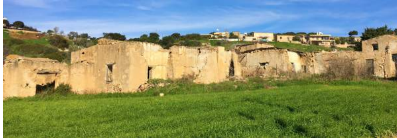
Figure 32: Collection of ruined buildings in the village
