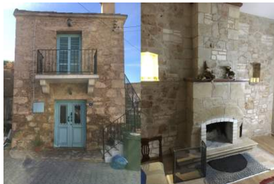
Figure 30: Exposed stone walls and the protected traditional appearance of the dwellings
