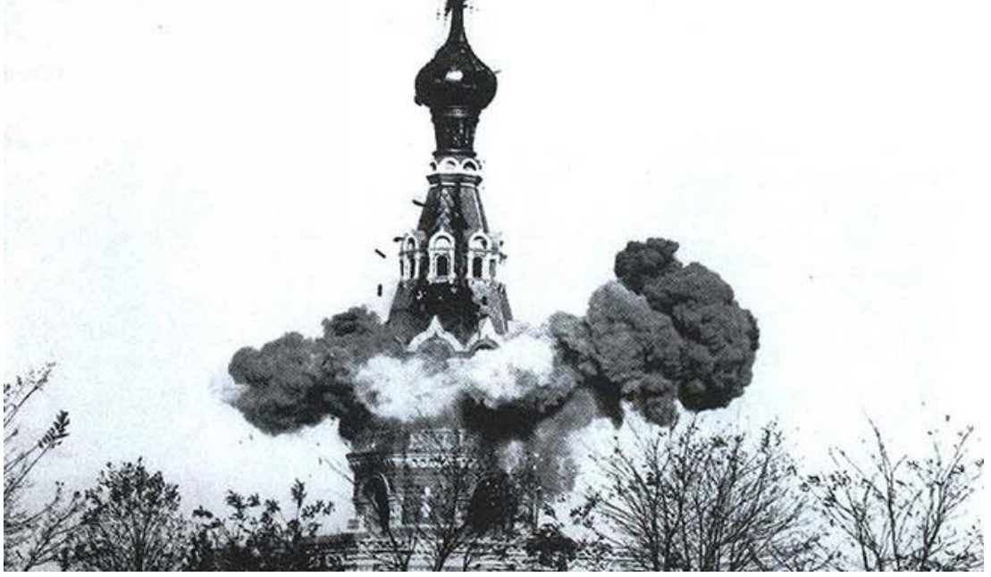
Figure 1: Demolition of the Monument at San Stefano
