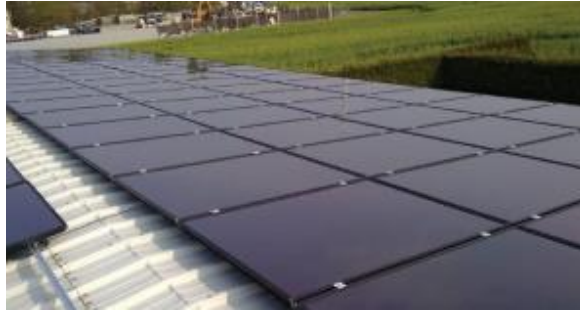
Figure 2.14: Cadmium Telluride Solar Cell (CdTe) Source: https://aplussolarsolutions.ca/what-are-thin-film-solar-panels/
