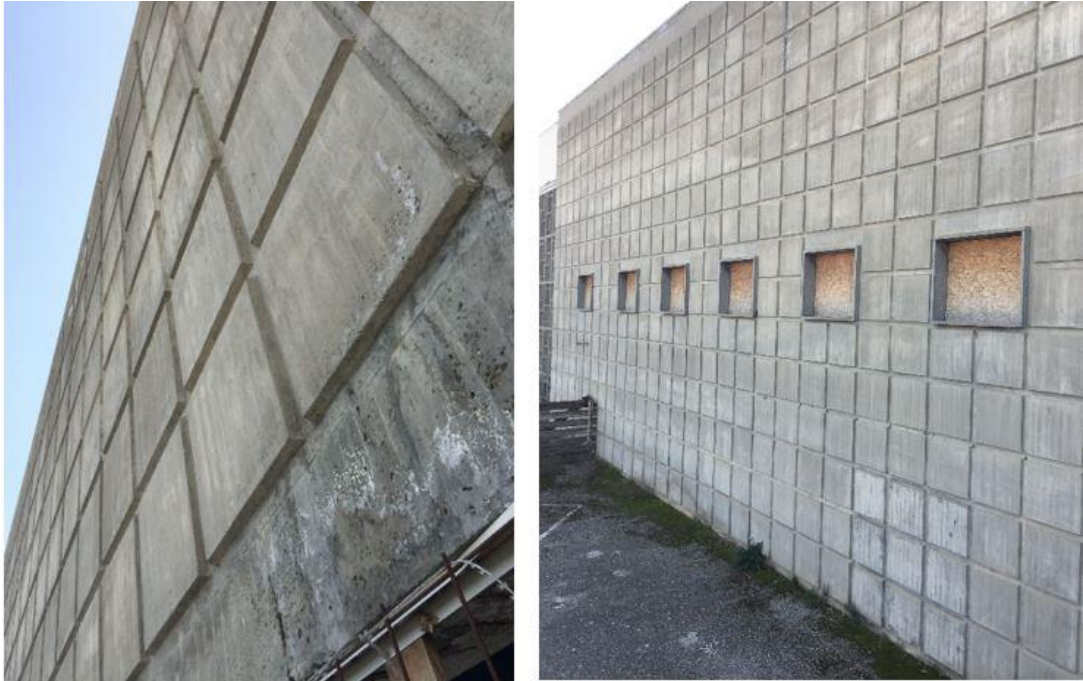
Figure 46: Photograph of NIAT Building- Concrete Façade Detailing (Photo: Abraşoğlu, M. 2022).
