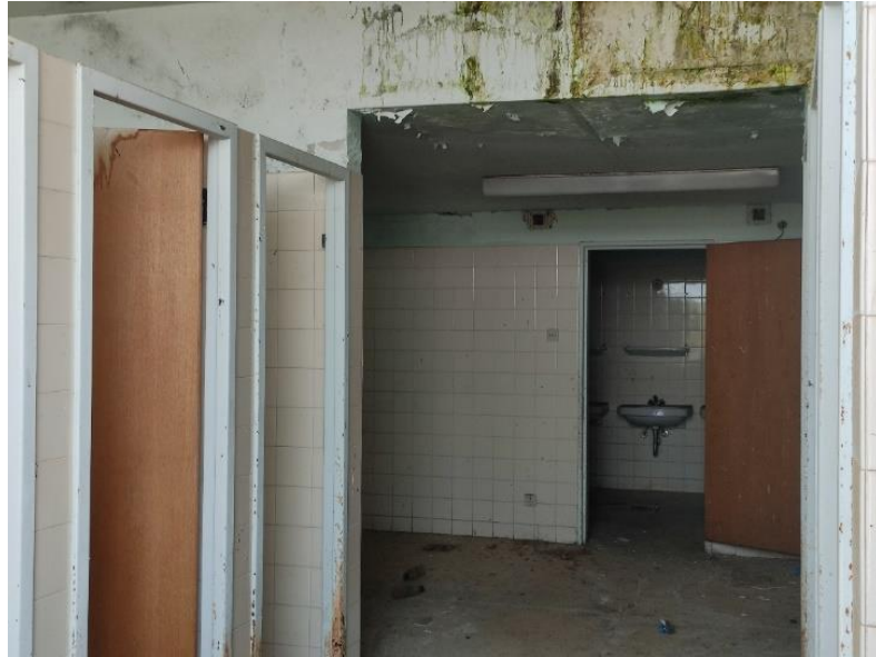
Figure 58: Wet Cores (Photo: Abraşoğlu, M. 2022).
