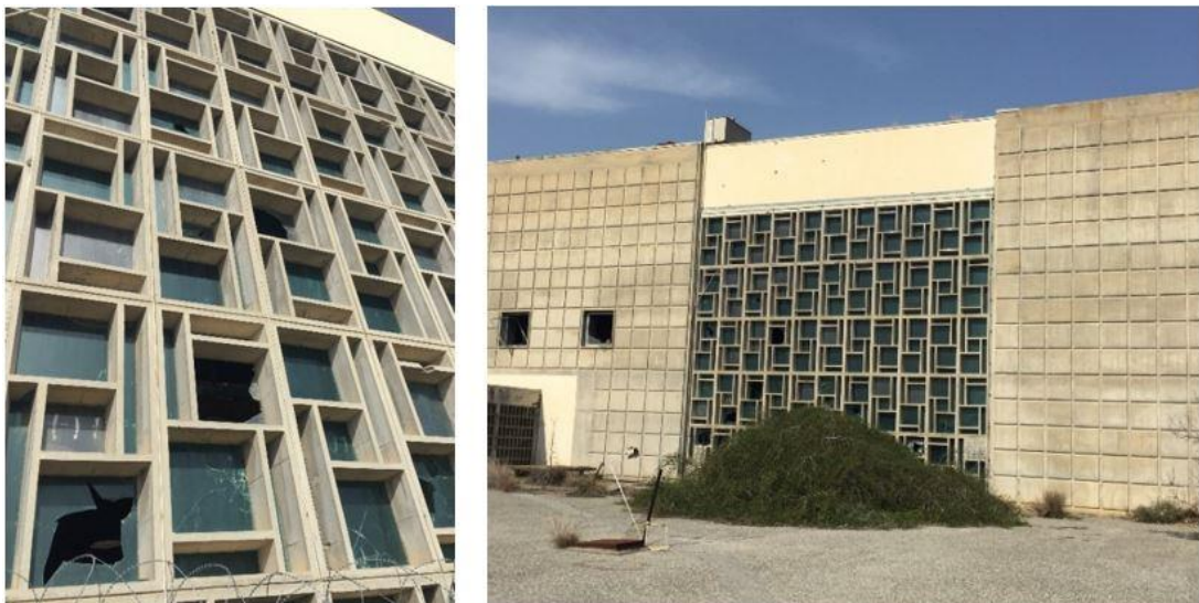
Figure 47: Photograph of NIAT Building- Concrete Façade Detailing (Photo: Abraşoğlu, M. 2022).
