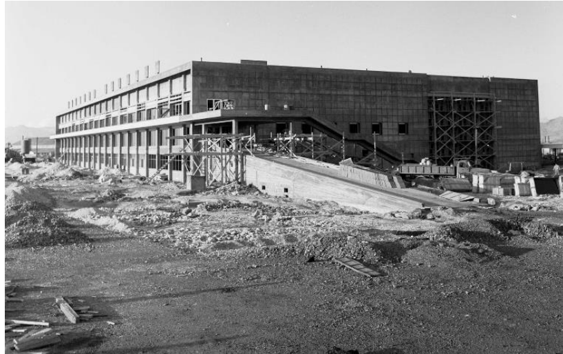
Figure 37: Photo of Construction of the New Terminal Building (The Republic of Cyprus Press and Information Office, Their Permission Granted, 2021).
