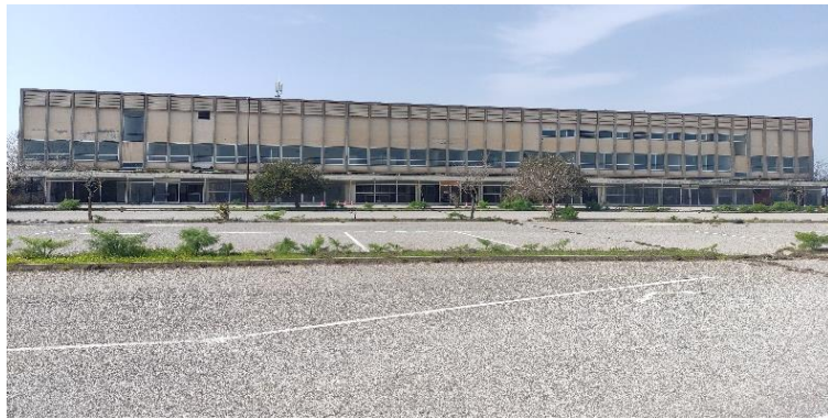
Figure 43: NIAT Building- View from Car Park (Photo: Türker, Ö. O. 2022).
