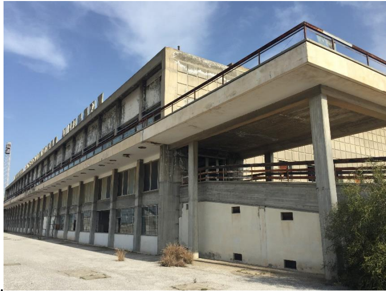
Figure 40: Photograph of Nicosia International Airport Terminal Building- View from Apron Showing the Send-Off Balcony (Photo: Abraşoğlu, M. 2022).
