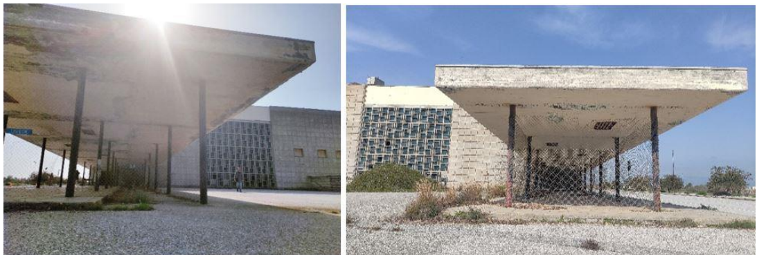
Figure 44: Photograph of NIAT Building- View of Drop-off Points- North- West Canopy, South East Canopy (Photo: Türker, Ö. O. 2022).
