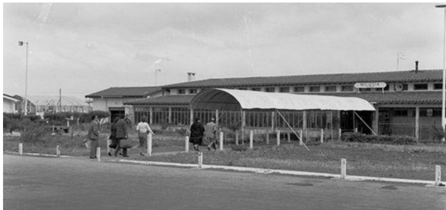
Figure 36: Enlarged Primary Terminal Building (URL 49).
