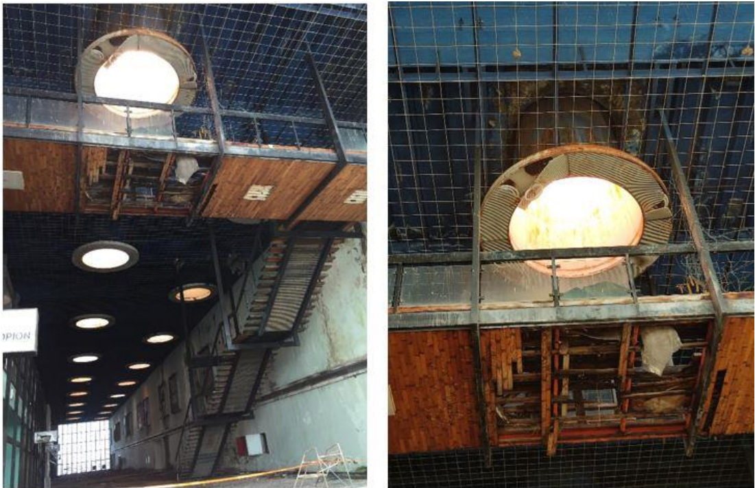
Figure 73: Skylights (Photo: Abraşoğlu, M. 2022).
