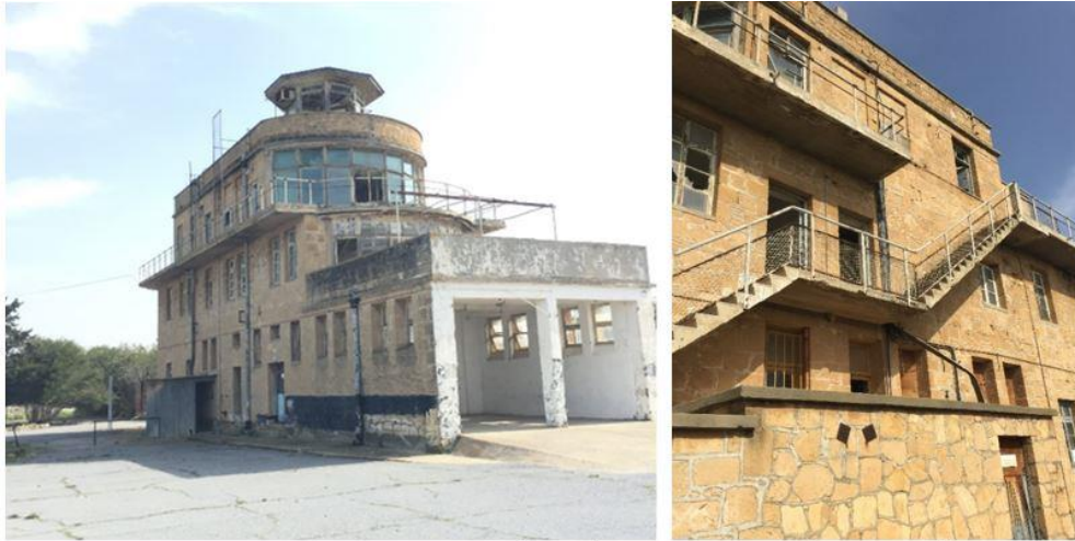
Figure 35: Photograph of Nicosia International Airport Old Control Tower (Photo: Abraşoğlu, M. 2022).
