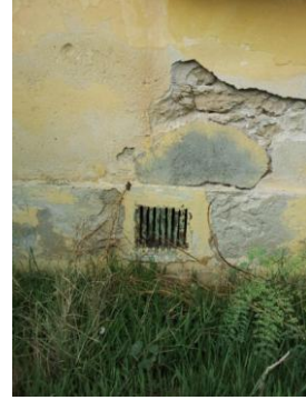
Figure V- 60: Ventilation hole for the wall and foundation in House 1 (Author, 2012)
