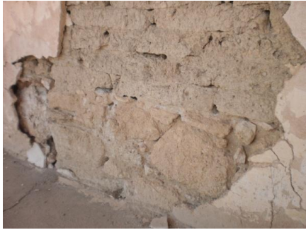
Figure V- 54: Adobe and stones in construction of wall in House 2 (Author, 2012)
