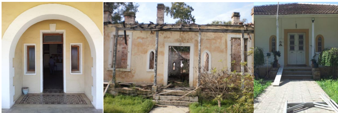
Figure V- 26: Entrance door and small windows in House 1, 3 and 4 (Author, 2012)
