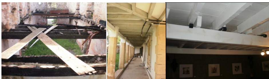
Figure V- 50: Timber floor views of House 3, 4 and 6 (Author, 2012)
