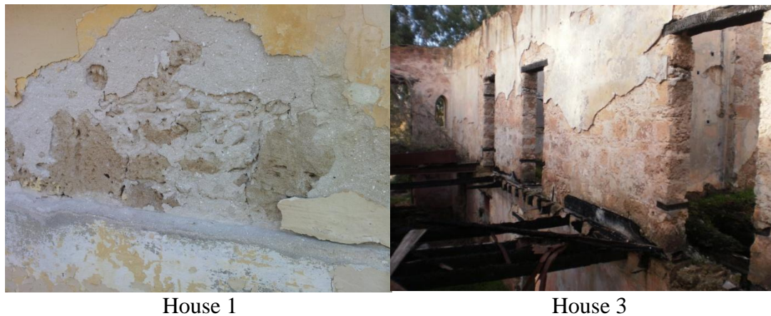
Figure V- 41: Visible yellow stone in the construction of walls (Author, 2012)
