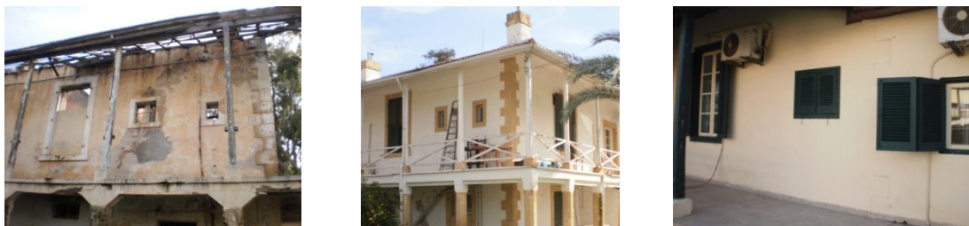
Figure V- 37: View of windows of service rooms in House 3, House 4 and House 5
