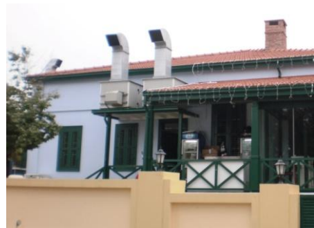
Figure V- 39: View of windows and toilet in House 6
