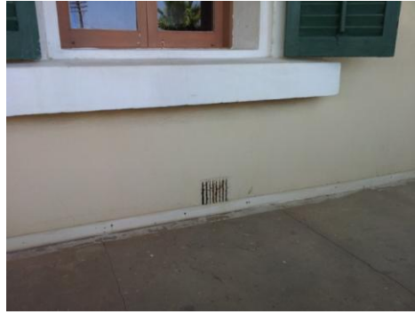
Figure V- 60: Ventilation hole for the wall and foundation in House 1 (Author, 2012)
