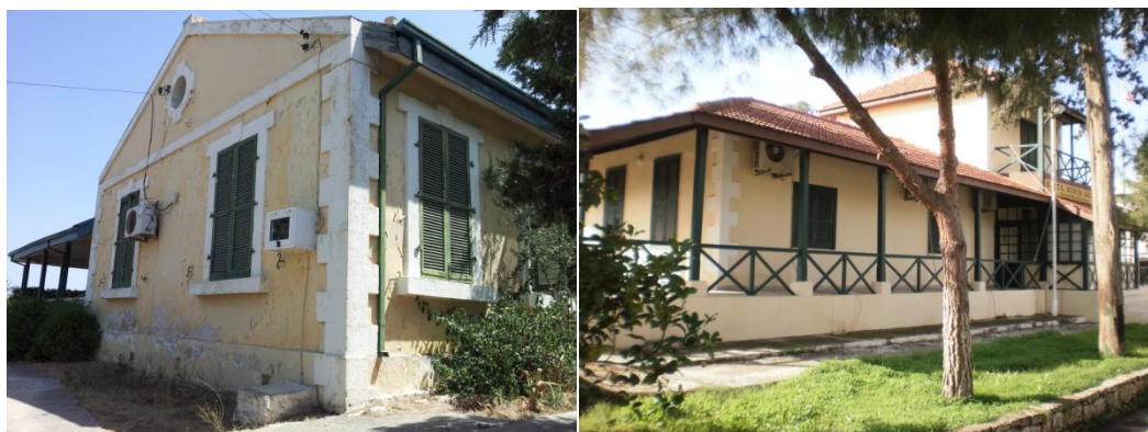
Figure V- 47: View of foundation level of House 1 and House 5 (Author, 2012)
