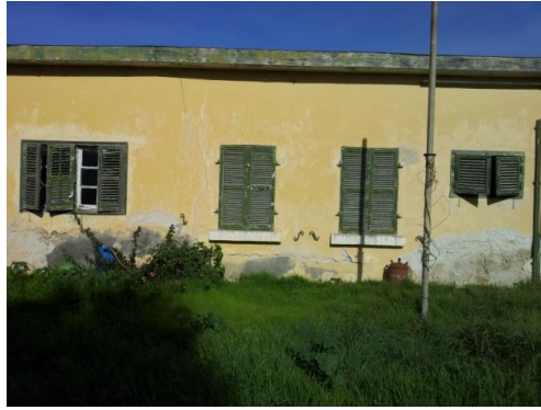
Figure V- 35: View of small windows of service rooms in House 1
