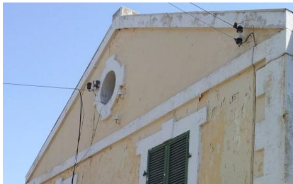
Figure V- 61: Ventilation hole for the roof in House 1 (Author, 2012)
