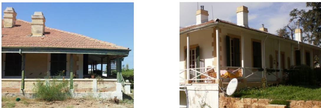
Figure V- 29: View of windows in House 1 and House 4 (Author, 2012)
