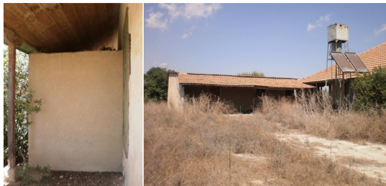
Figure V- 7: View of added and re-constructed part of House 2 (Author, 2012)
