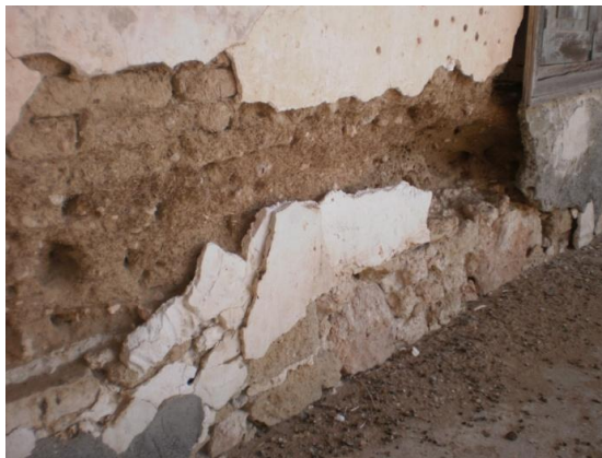
Figure V- 43: Visible adobe (mud-brick) and small round fieldstones under it (Author, 2012)
