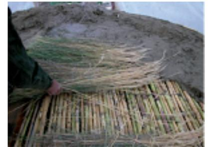
*Laying down the roof with cane, saddle grass and mud*
