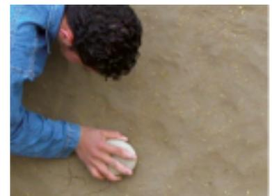
*Beating down the render cracks on the wall*
