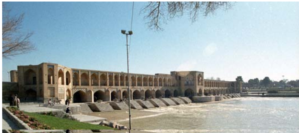
Figure 33: Khajoo Bridge, isfahan, Photo: Rafooneh M.Sani
