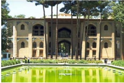
(Hasht Behesht palace, photo: http://archnet.org/library )
