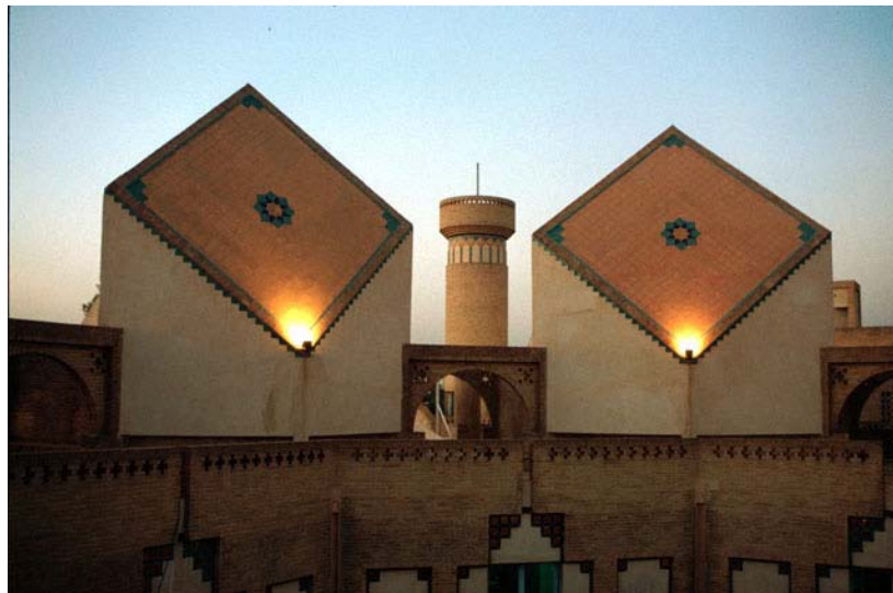
Figure 118: Dezful cultural center, View to roof structure, Photo: http://www.archnet.org
