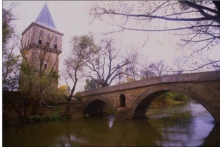
Figure 37: Fatih Bridge over Tunca near Edirne, Turkey, Photo: Ustun Alsac photo collection
