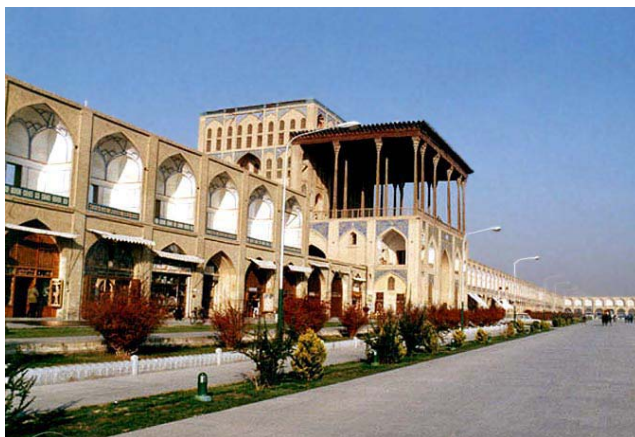
Figure 104: The contrast between light and mass structure, Aliqapu palace, Isfahan,
