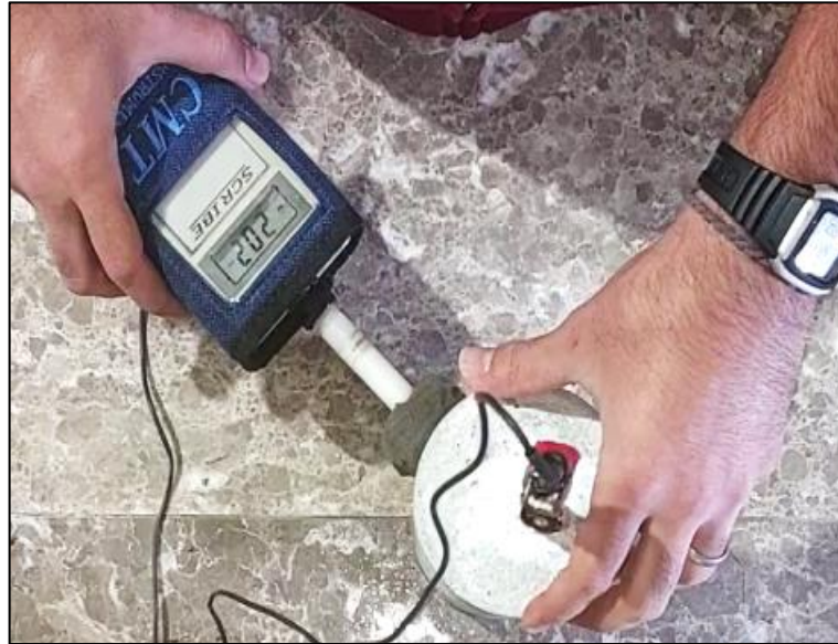
Figure 11: Half-cell potential test equipment
