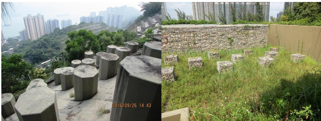
Figure 2: Baffles used in Hong Kong to mitigate debris flow disaster in conjunction with a rigid barrier (Yang et al., 2021)
