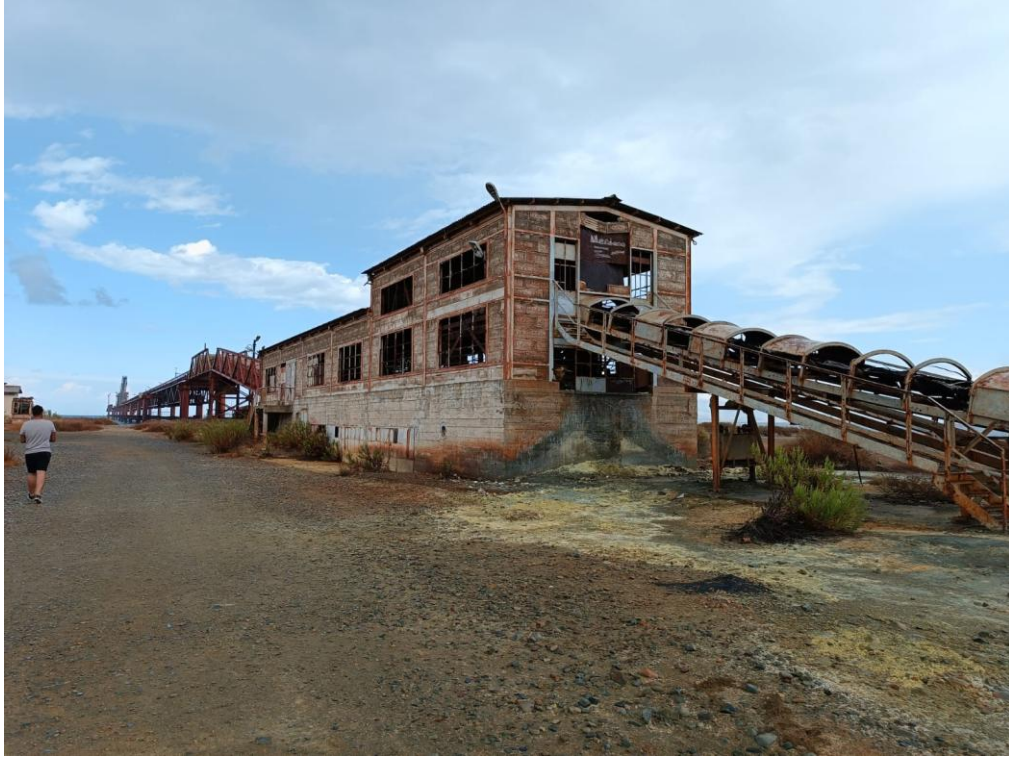
Figure 8: View of The CMC Mine Loading Deck From The Northwest, Showing Structural Features and Environmental Context. (Photo by Author, 2024)
