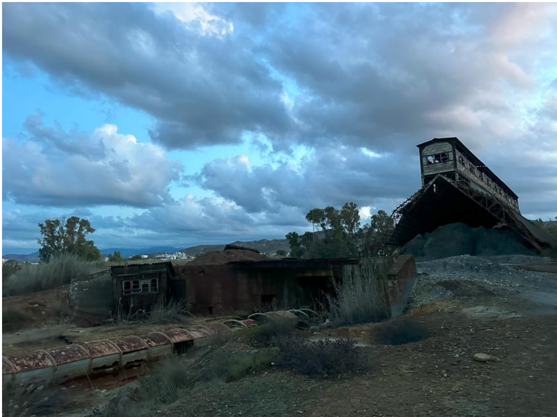
Figure 11: View of The CMC Mine Loading Deck From The Northwest, Showing Structural Features and Environmental Context. (Photo by Author, 2024)
