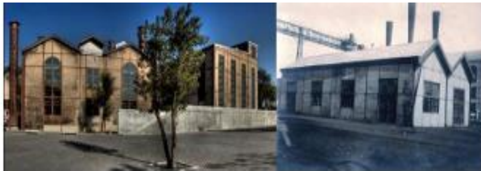
Figure 5: Adaptive Reuse in Santralistanbul Previous and New Building. (Photos by Sudjic, D Hussein, N. (2021))
