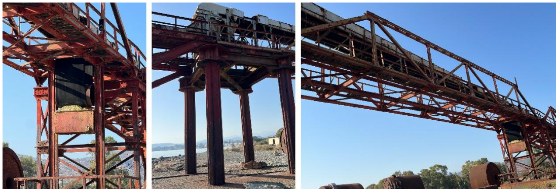
Figure 15: Steel Loading Bridge (Photo by Author, 2024)
