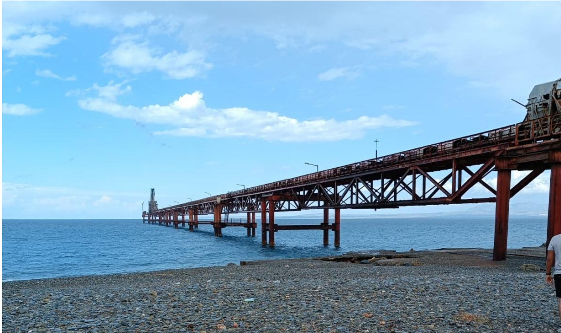
Figure 23: View of The CMC Mine Loading Deck From The Northwest, Showing Proposed Ancient Heritage Gallery Area. (Photo by Author, 2024)
