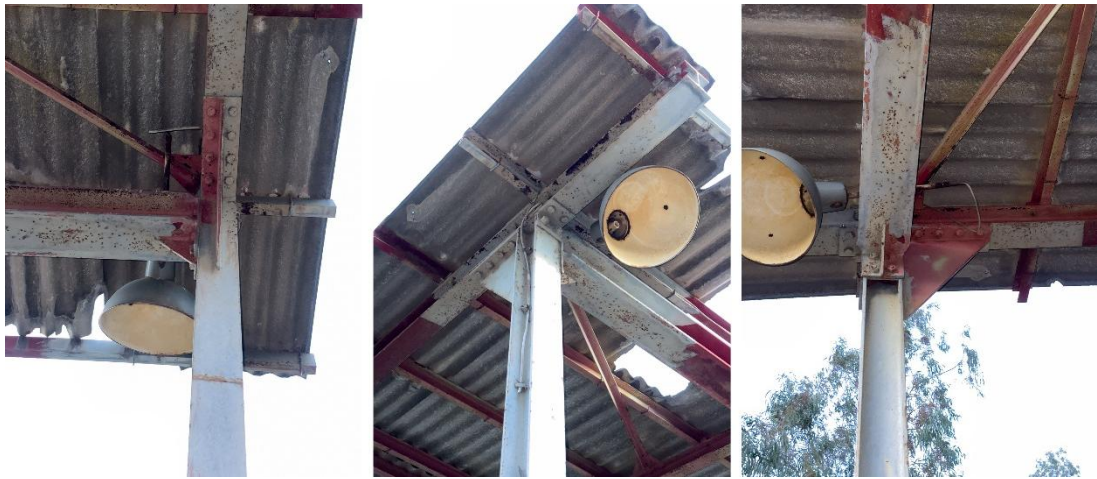
Figure 14: Steel Connections & Decays (Photo by Author, 2024)
