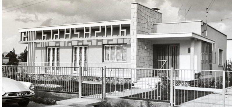
Figure 62: The original design of Niyazi Ali House with single floor, 1961 (from Abdullah Onar archive with the permission of Anber Onar)
