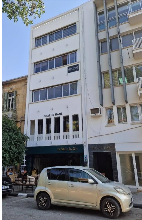
Figure 47: Onar Office Block, Nicosia, 1974 (photo taken by the author)
