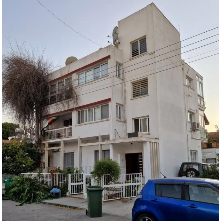
Figure 67: Today's appearance of Adnan Tahsin House with the additional floors (photo taken by the author)
