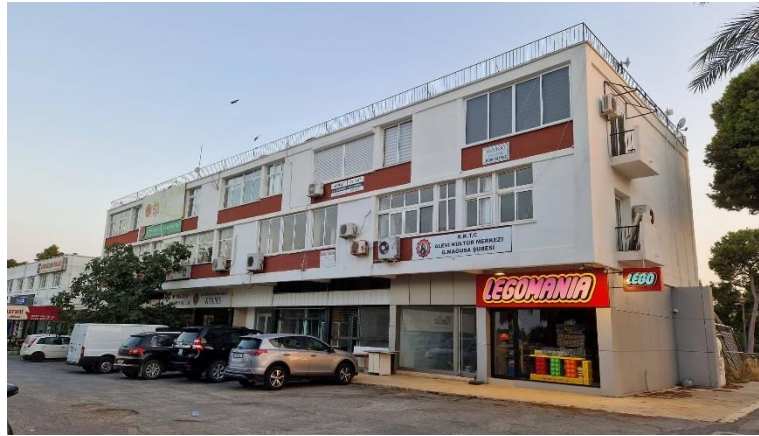
Figure 45: Evkaf building in Famagusta by Abdullah Onar in 1957 (photo taken by the author)
