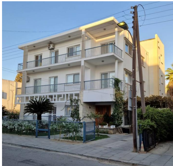
Figure 63: Today's appearance of Niyazi Ali House with the additional floors (photo taken by the author)
