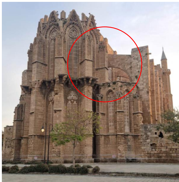
Figure 4: Flying buttresses of St. Nicholas Cathedral (photo taken by the author)
