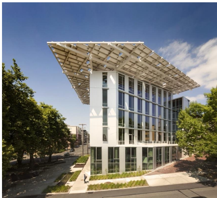
Figure 4:Bullitt center: found in seattle usa (URL 3)
