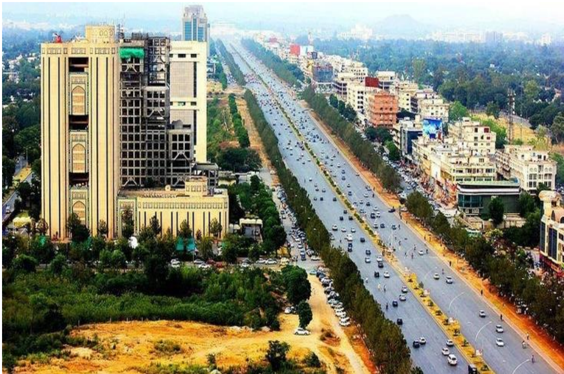
Figure 3: Aerial view of blue rea (from google images)
