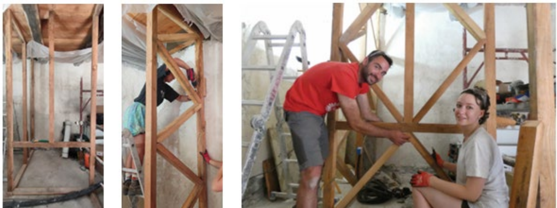
Figure 37: Beginning of the wall construction, FoRTI, 2023
