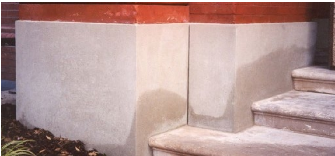
Figure 6: Final patching repair (URL3)
