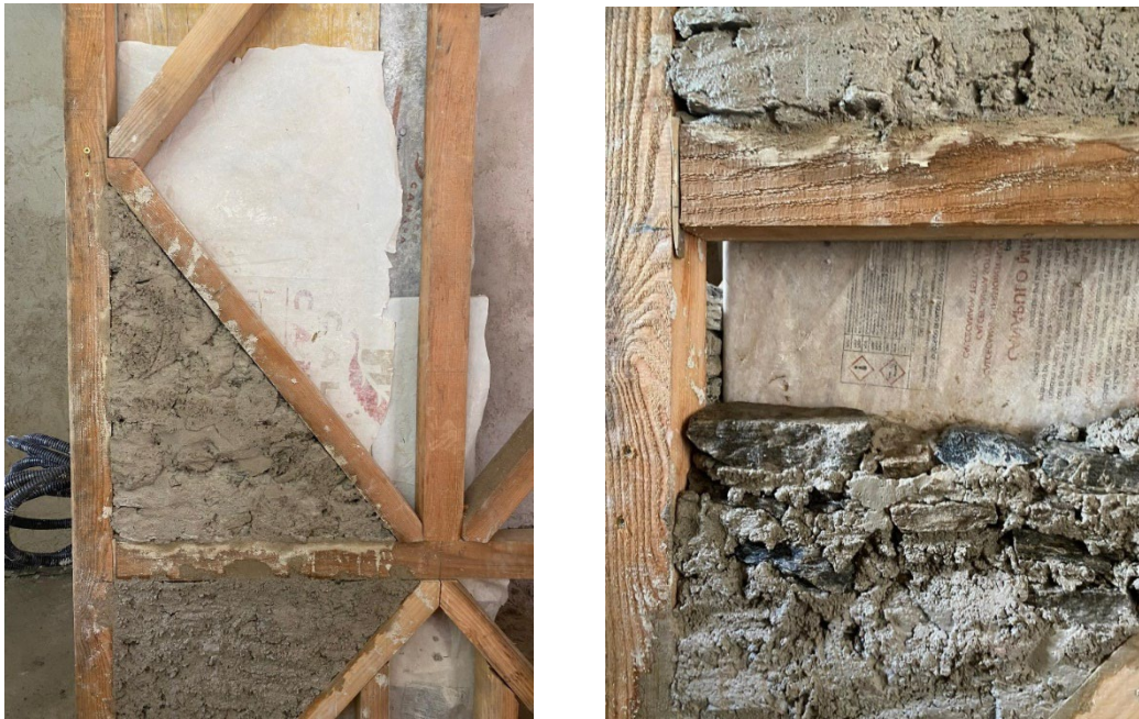
Figure 38: Stone wall filling, photo by author, Ghesc, Italy, 2023
