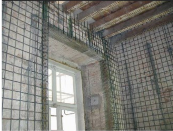
Figure 3: Masonry wall from the inside with steel mesh (Meireles & Bento, 2013, p:11)
