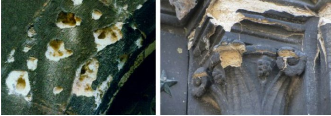
Figure 16: Examples of black crusts in limestone (Rodrigues, 2015, p:270)
