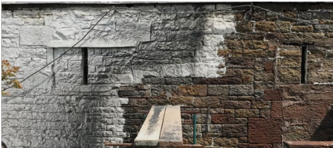
Figure 4: Stone and brick sandblasting (URL2)
