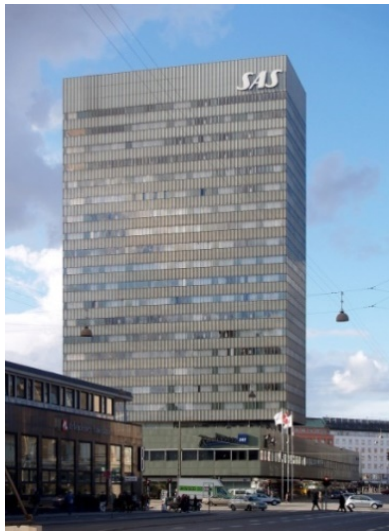
Figure 20: Facade of the Radisson Hotel (Seier, 2008)
