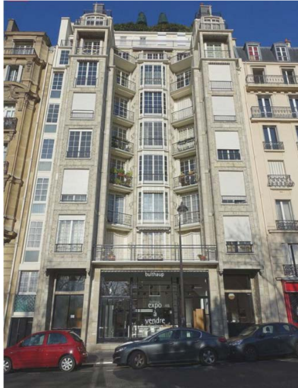
Figure 6: Reinforced Concrete Apartment, Auguste Perret, Paris, 1903 ( https://en.wikipedia.org/wiki/Auguste_Perret )
