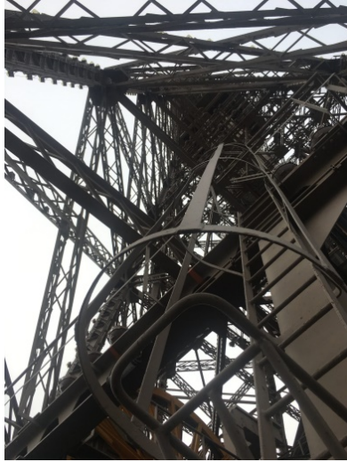
Figure 3: Steel work of Eiffel Tower (Öztürk,2018)
