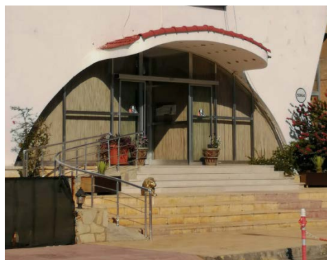
Figure 51: Entrance door with arch frame in Golden Plage Hotel
