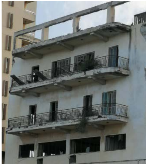
Figure 39: Florida Hotel timber shutters and iron railing
