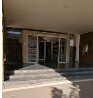
Elevated door with staircase in Golden Sands Hotel
