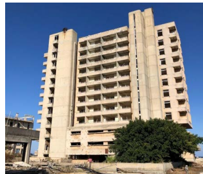
Figure 34: Rectangular shaped facade of Aspelia Hotel
