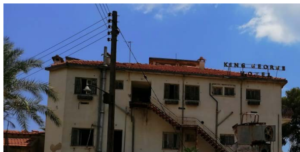
Figure 53: Slopped roof in King George Hotel
