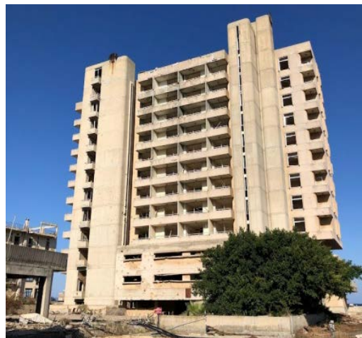
Figure 44: Strip balconies in Aspelia Hotel
