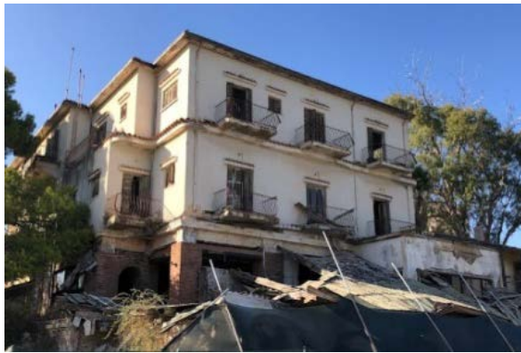
Figure 47: Low rise hotel buildings (King George Hotel)
