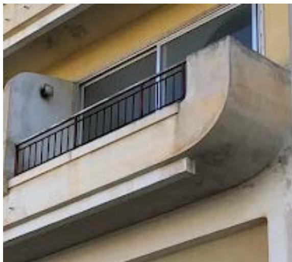
Figure 48: Eave of balcony in Arcadian Hotel
