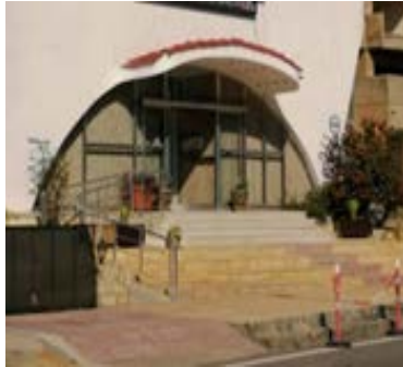
Arch frame doorway in Golden Plage Hotel
