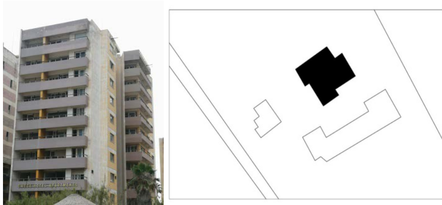
Figure 36: Cubic shaped facade with attachments in Omega Hotel Apartment
