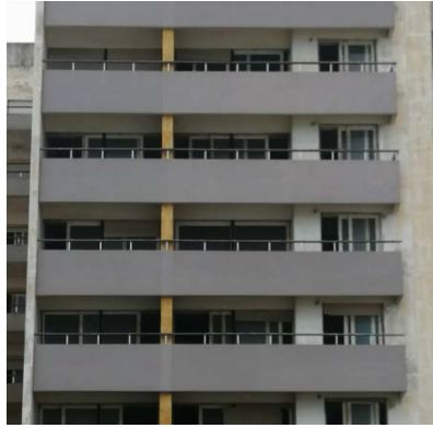
Figure 49: Horizontal element as a balustrade in Omega Hotel Apartment
