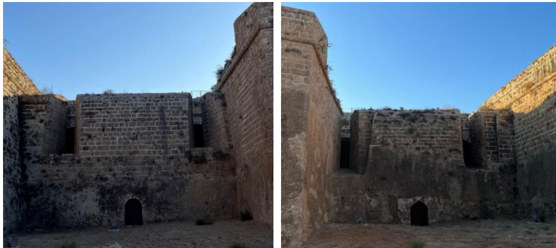
Figure 65: The Martinengo Bastion Side Entrances to Bateria (Author)
