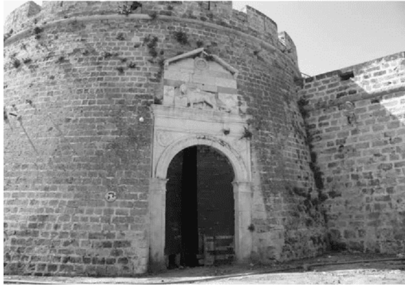
Figure 57: Nicolo Priuli, The Sea Gate Bastion, Famagusta, 1496 (Langdale, 2010)
