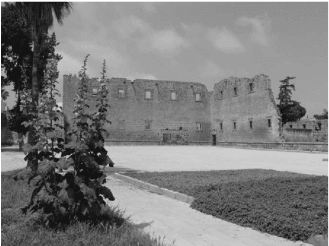
Figure 71: Palazzo Del Provveditore, Famagusta, Walls of Residential Block and Cortile (Langdale, 2010)
