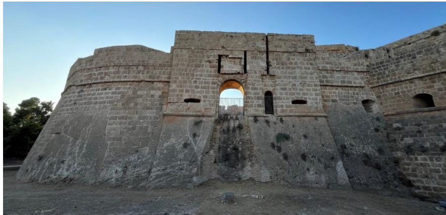
Figure 59: The Ravelin Bastion Old Entrance (Author)
