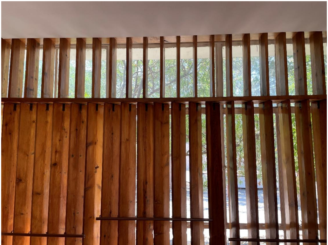
Figure 74: Photograph of the sun breaker and its handles in the daily living room taken by the author
