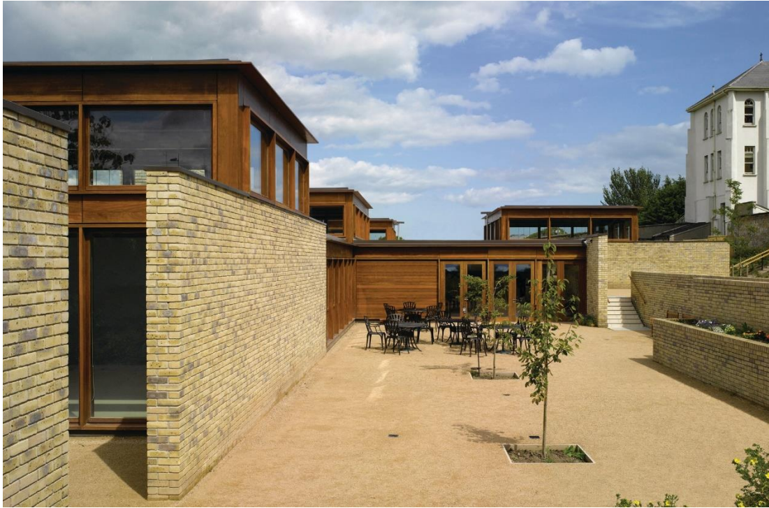
Figure 15: Facade of Alzheimer's Respite Centre [94]
