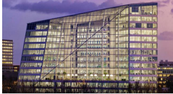
Figure 17: The Edge Building in Amsterdam (PLP Architecture, n.d.).
