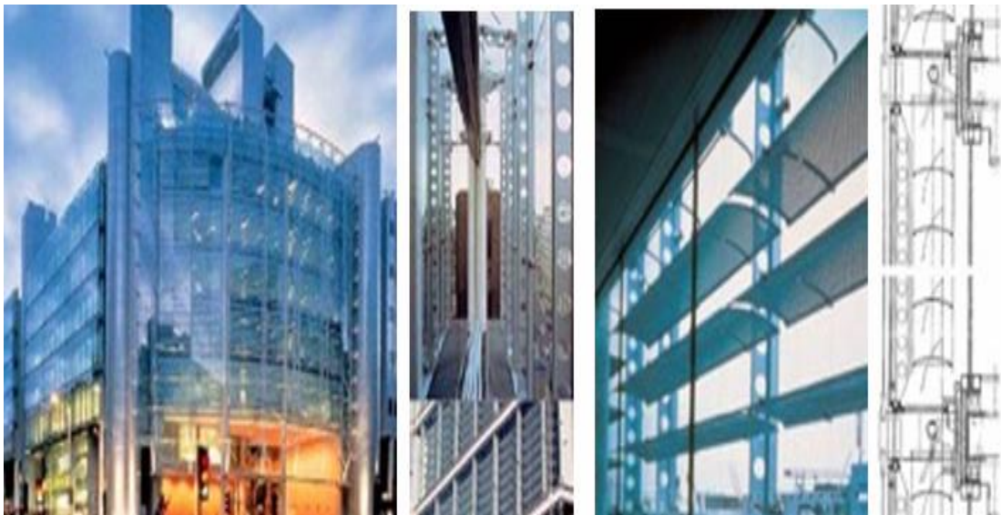
Figure 10: Example of Multi Storey Double-Skin Façade System (Sharma, 2003 As Cited In Boduroğlu & Seçer Kariptaş, 2010).
