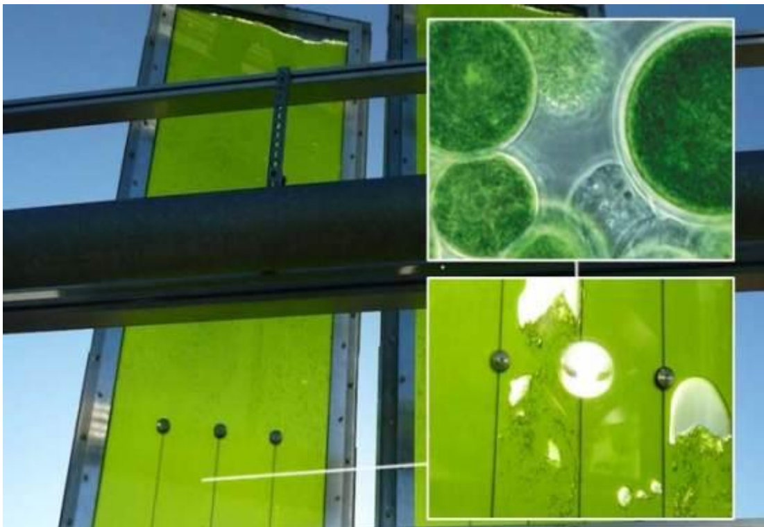
Figure 36: Microalgae-Filled Photobioreactor Panel Providing Dynamic Shading and Energy (Beciri, 2013).
