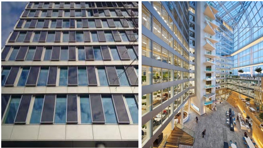
Figure 28: Solar Pv Panels on The South Side and Atrium (PLP Architecture, n.d.).
