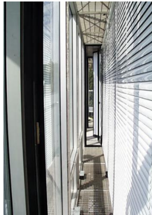
Figure 22: Venetian Blinds Installed in The Cavity Between Glazing Layers (Loncour Et Al., 2005).
