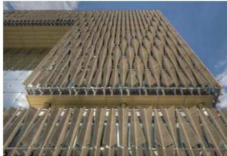
Figure 21: Solar Control System on The Exterior Face of The Building Skin (Radwan, 2017).
