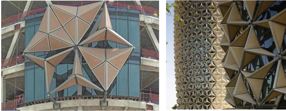
Figure 16: Al Bahar Towers. Dynamic Facade Modules with Integrated Light, Wind, and Rain Sensors for Real-Time Environmental Response. (Karanouh & Kerber, 2015).
