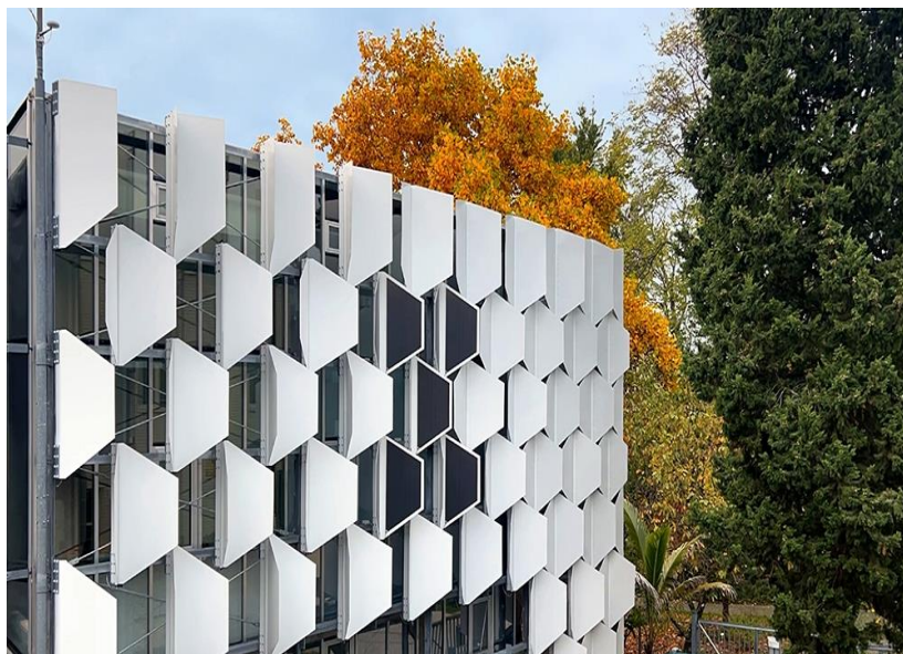
Figure 39: Front View of Flectoline Façade with Semi-Closed Modules (University of Stuttgart, Institute of Building Structures and Structural Design, 2024).
