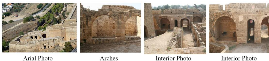
Figure 4.9: Ravelin/Land Gate (UNDP-PFF Ravelin/Land Gate project, 2018)
