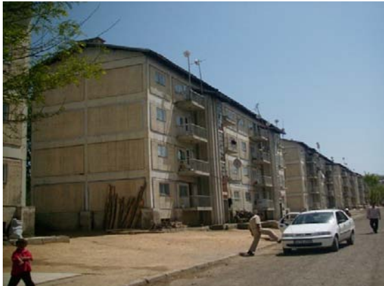
Fig. 2 Bingöl earthquake houses [6].
