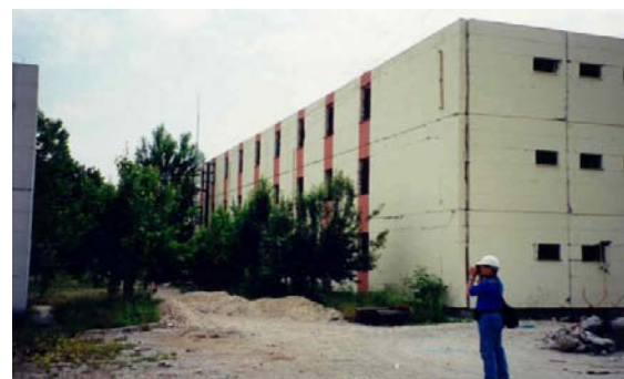
Fig. 5 Dormitory building in Bolu.
